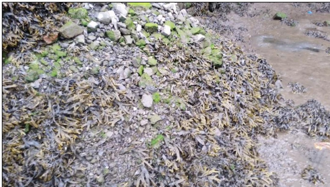
Plate 2: Substrate immediately adjacent to Martins Quay wall (unsuitable for aquatic QI species of the Natura 2000 Sites).
